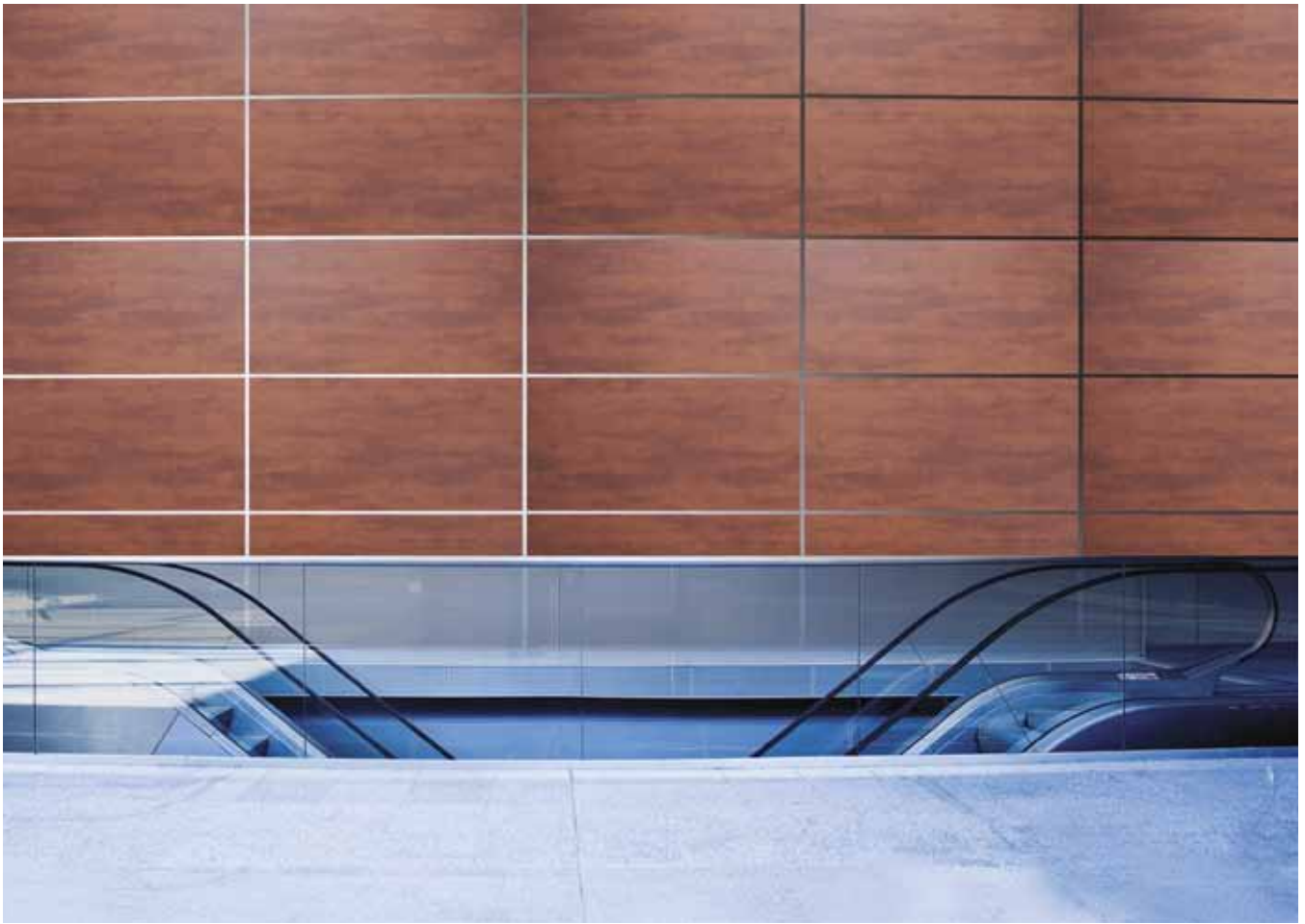
Chemetal #600 Weathered Aluminum as wall panels, public space.
